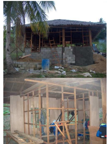
Halfway done school dormitory
