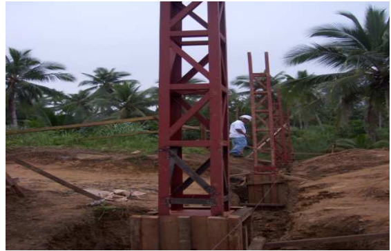
Building columns finally erected after successive heavy rains
